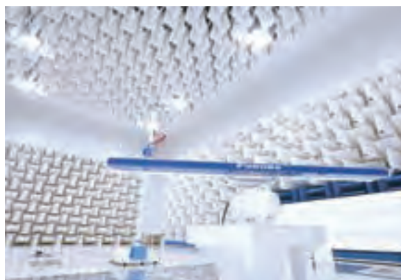
In-house EMC* testing environment
